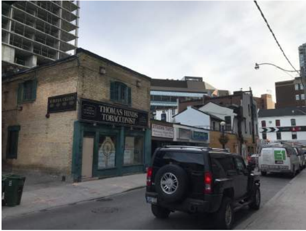
Site of Eight Cumberland Condos, Cumberland Street properties
