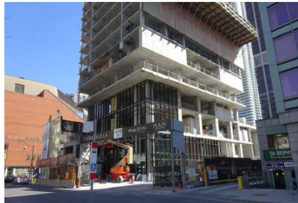
1 Yorkville, under construction, looking southwest
