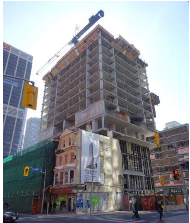
1 Yorkville, under construction, looking southwest
