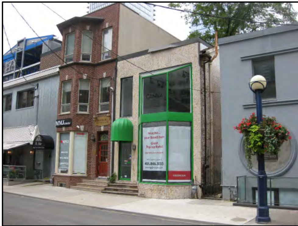
Photograph 8: View of 18 and 20 Cumberland Street, looking northwest (October 11, 2017).
