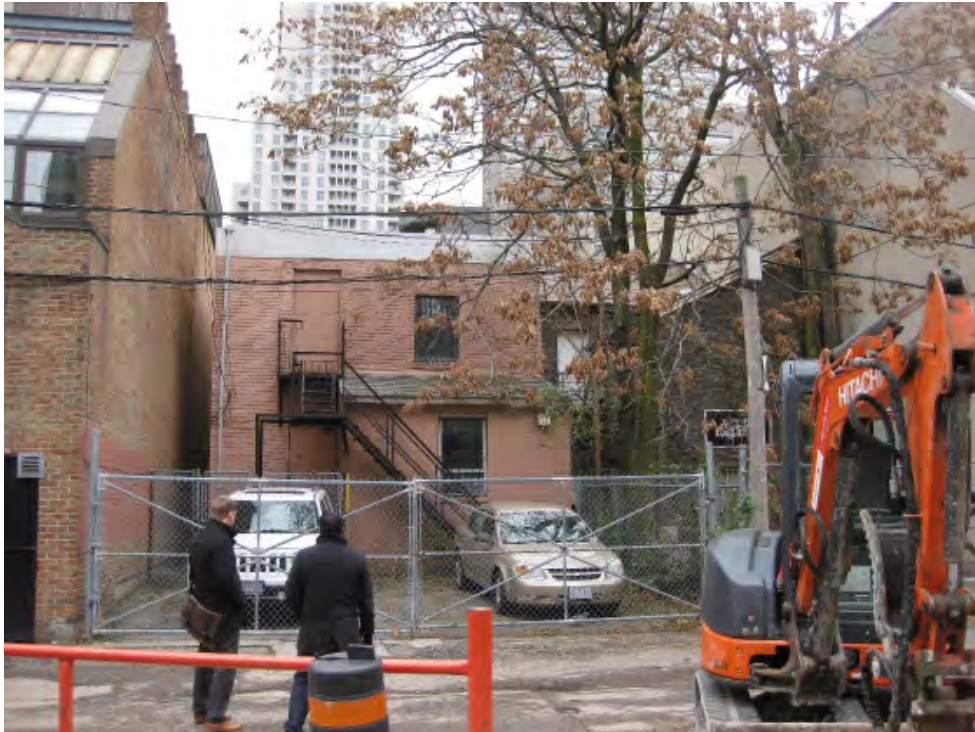
Photograph 19: View of the north face of 16 Cumberland Street, looking south (November 14, 2017).
