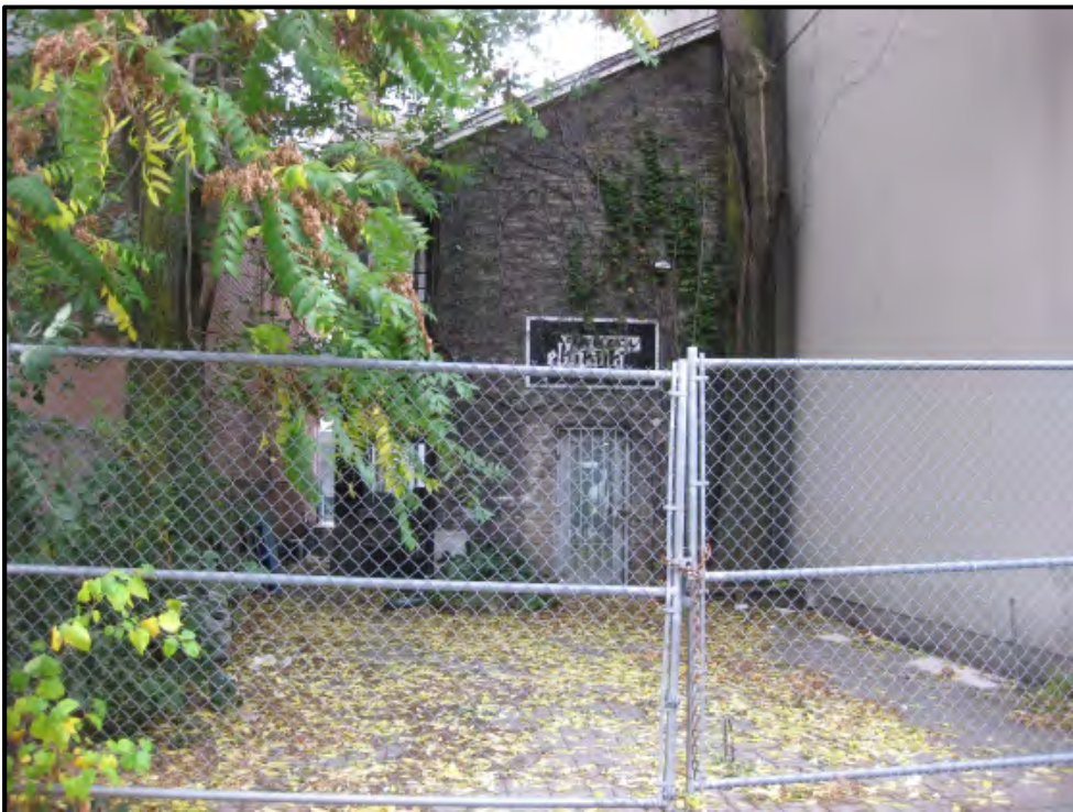
Photograph 20: View of the south face of 18 Cumberland Street, looking south (October 11, 2017).
