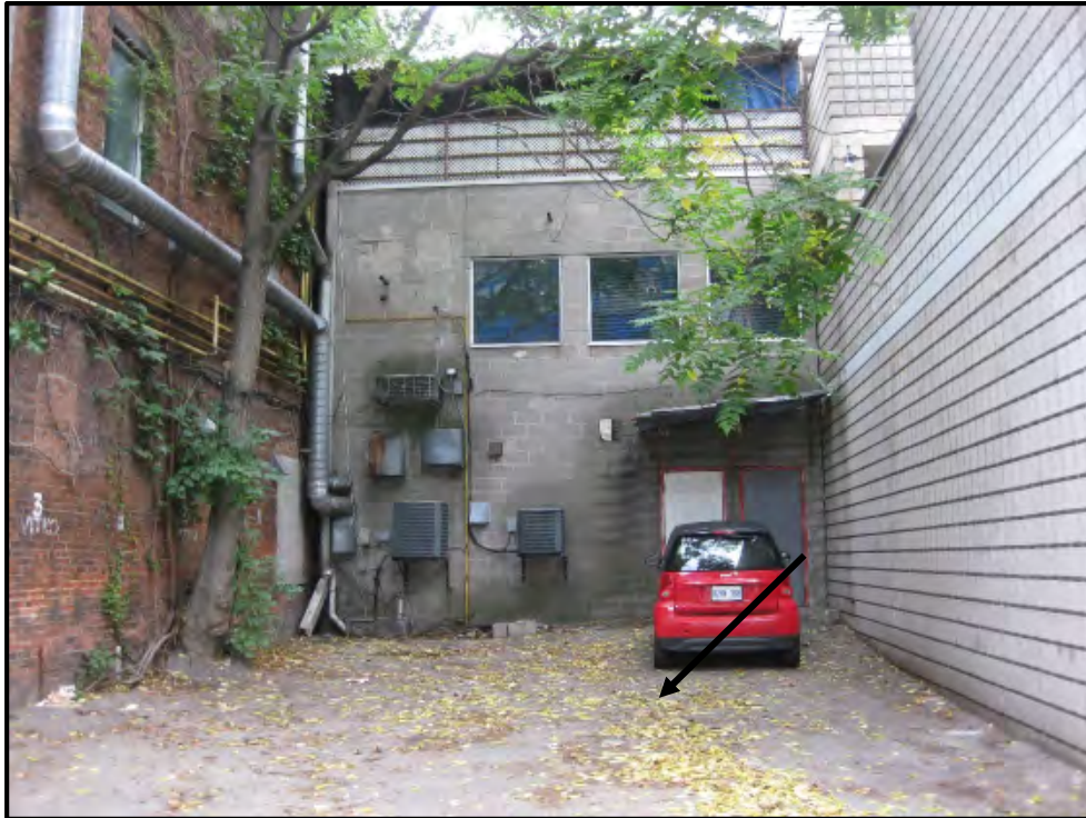
Photograph 17: View of the south face of 19 Yorkville Avenue, looking north (October 11, 2017). The approximate location of a previously installed monitoring well is indicated by the arrow.
