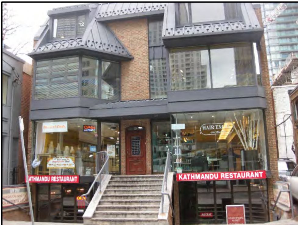
Photograph 6: View of 12 and 14 Cumberland Street, looking north (November 14, 2017).
