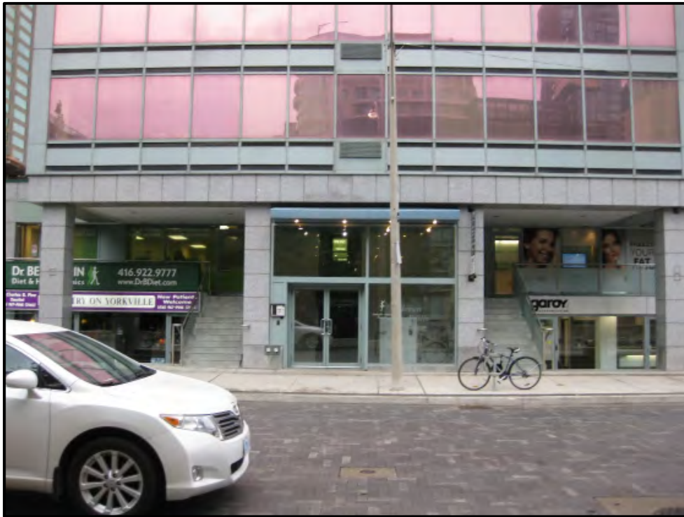
Photograph 3: View of the ground level of 11 Yorkville Avenue, looking south (October 11, 2017).
