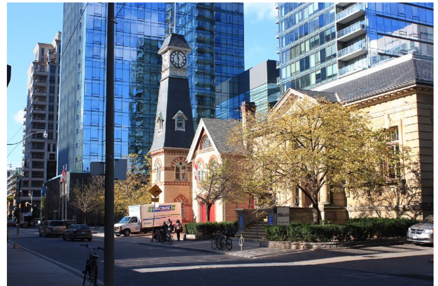
Looking west along the north side of Yorkville Avenue. The low-rise brick buildings visible in the photograph are listed in the Heritage Register: the Northern Branch Toronto Public Library (22 Yorkville) and Fire Hall #10 (34 Yorkville). Note the Four Seasons Hotel and Residences in the background.
