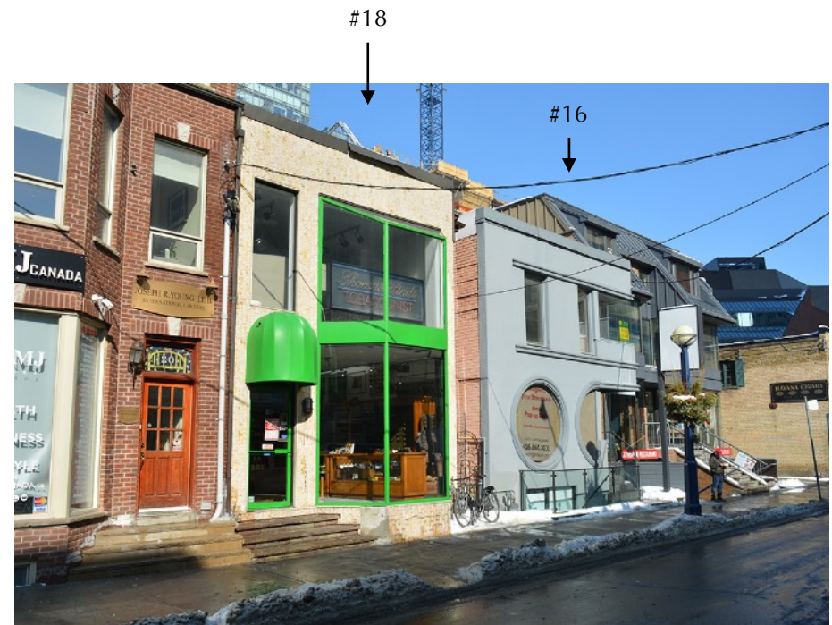
Photograph above, taken in 2018, is a similar view as the 1961 photograph on the left. 16 and 18 Cumberland Street are identified with arrows. In the late 20th century, the buildings at 16 and 18 Cumberland were altered unrecognizably (annotations by GBCA Architects).
