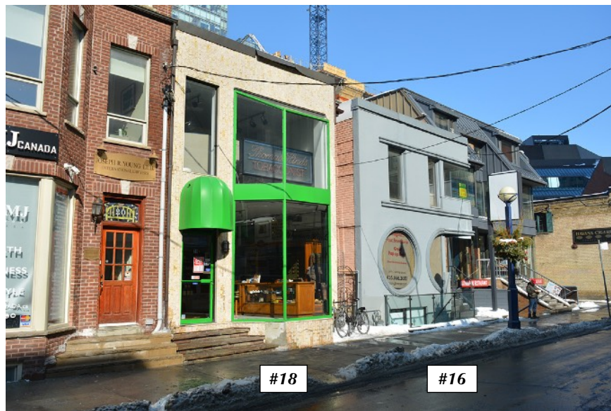
Looking along the north side of Cumberland Street, towards the two subject buildings on the development site. 16 Cumberland is currently vacant and 18 Cumberland is occupied by a commercial tenant.
