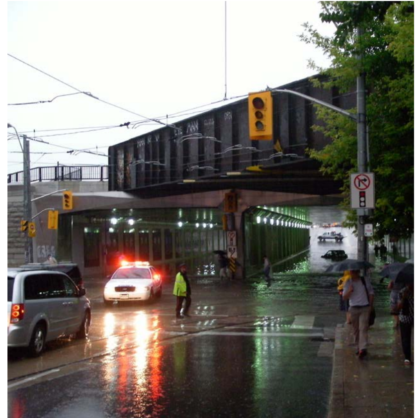
Figure 11: The immediate importance of resilient design was demonstrated in Toronto by the 2013 flooding of downtown streets and buildings (Courtesy of user:Eastmain / Public Domain)
